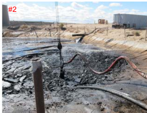
Picture #2 depicts hazardous accumulation on a sludge pond. Sludge ponds are designed to separate oil from produced water waste prior to discharge into a pond; however, this sludge pond appears to be overrun with oil accumulation.
