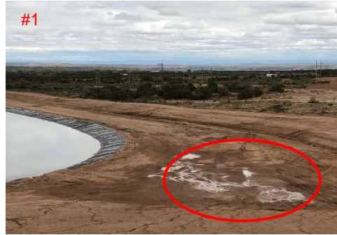
Picture #1 shows evidence of exploration and production water waste leaking from an evaporation Pond, which should never happen.
