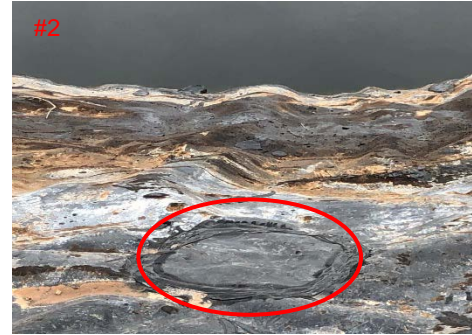
Picture #2 depicts a patch that was used to fix a hole in the liner of an evaporation pond where leaking occurred.
