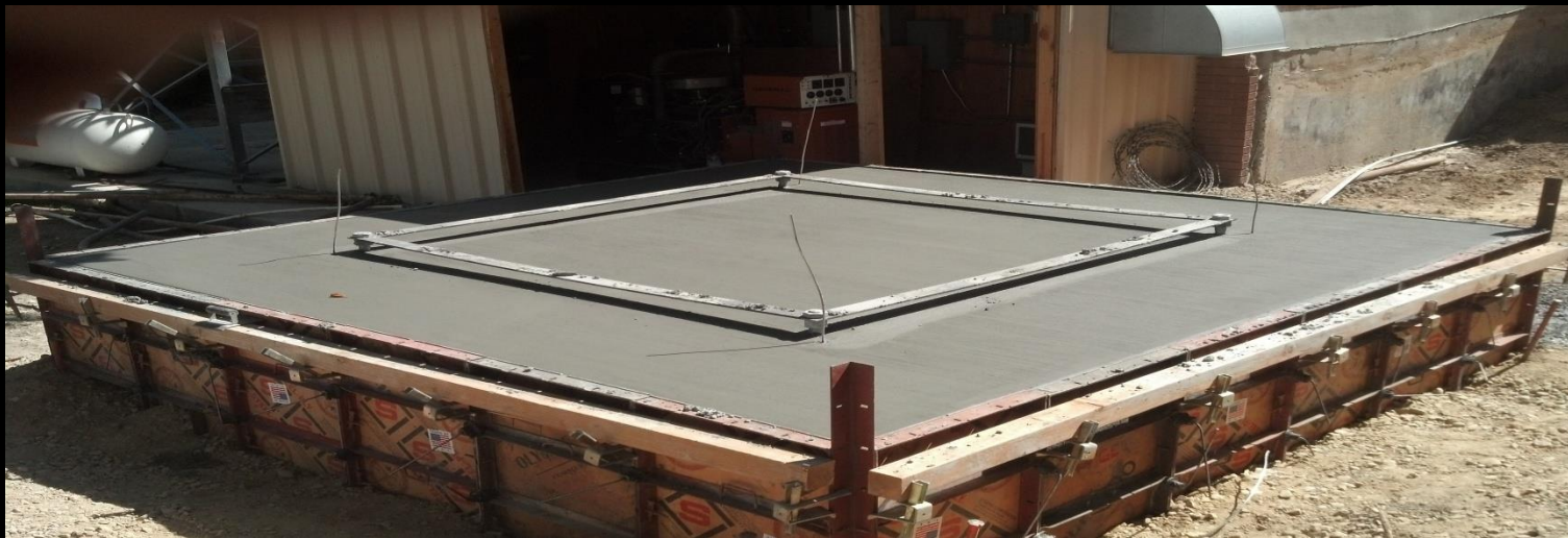
New Tower Footer for Price Dispatch Center
