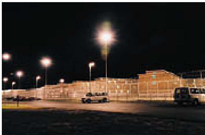
Figure 4.4: Typical nighttime fence line illumination level of 2-3 foot candles.
