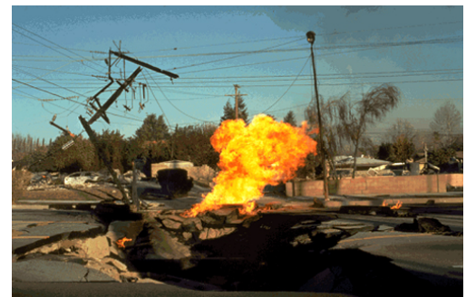
Figure 1.2: Natural Gas Line Ruptured by Liquefaction in Grenada Hills CA, 1994
