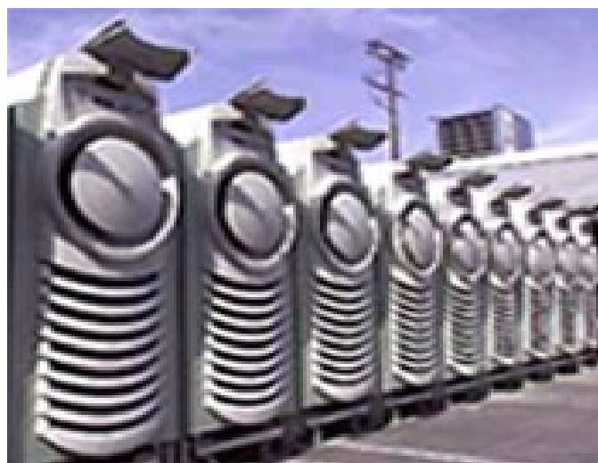
Figure 4.15: Multiple 500 kW micro-turbines connected in a staged parallel arrangement
