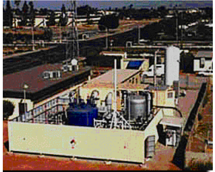
Figure 4.9: A Test Fuel Model Cell Cogeneration Plant at Miramar Naval Air Station
