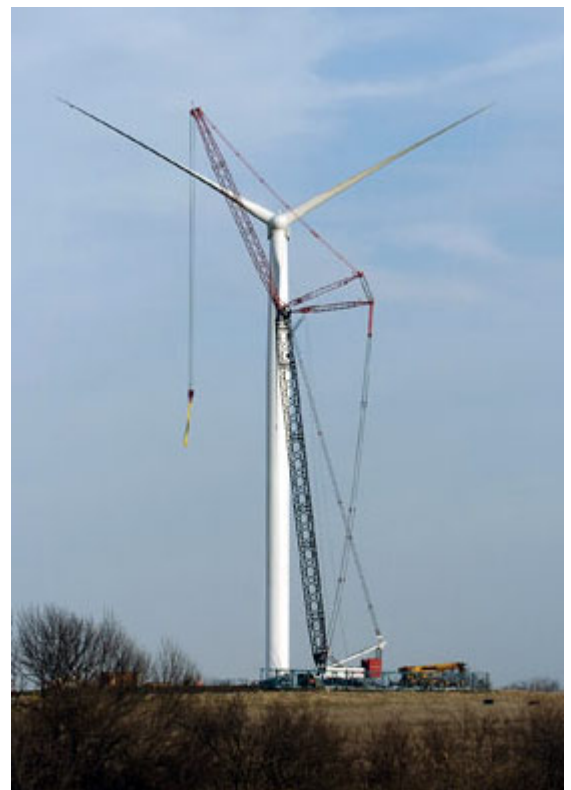
Figure E.1: Large Suzlon Wind Turbine Installation
