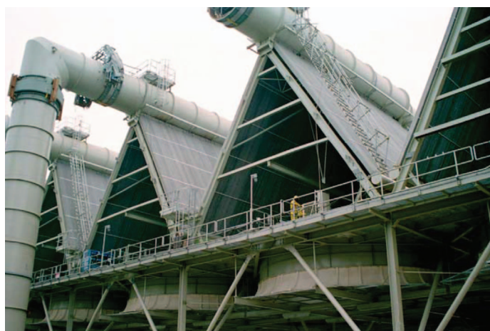
Figure 4. Air-cooled condenser showing horizontal cooling fans and heat exchanger tubes
