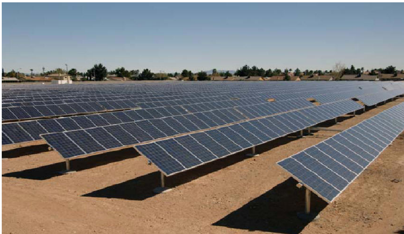
Figure E.2: Racked/Angled PV Panels
