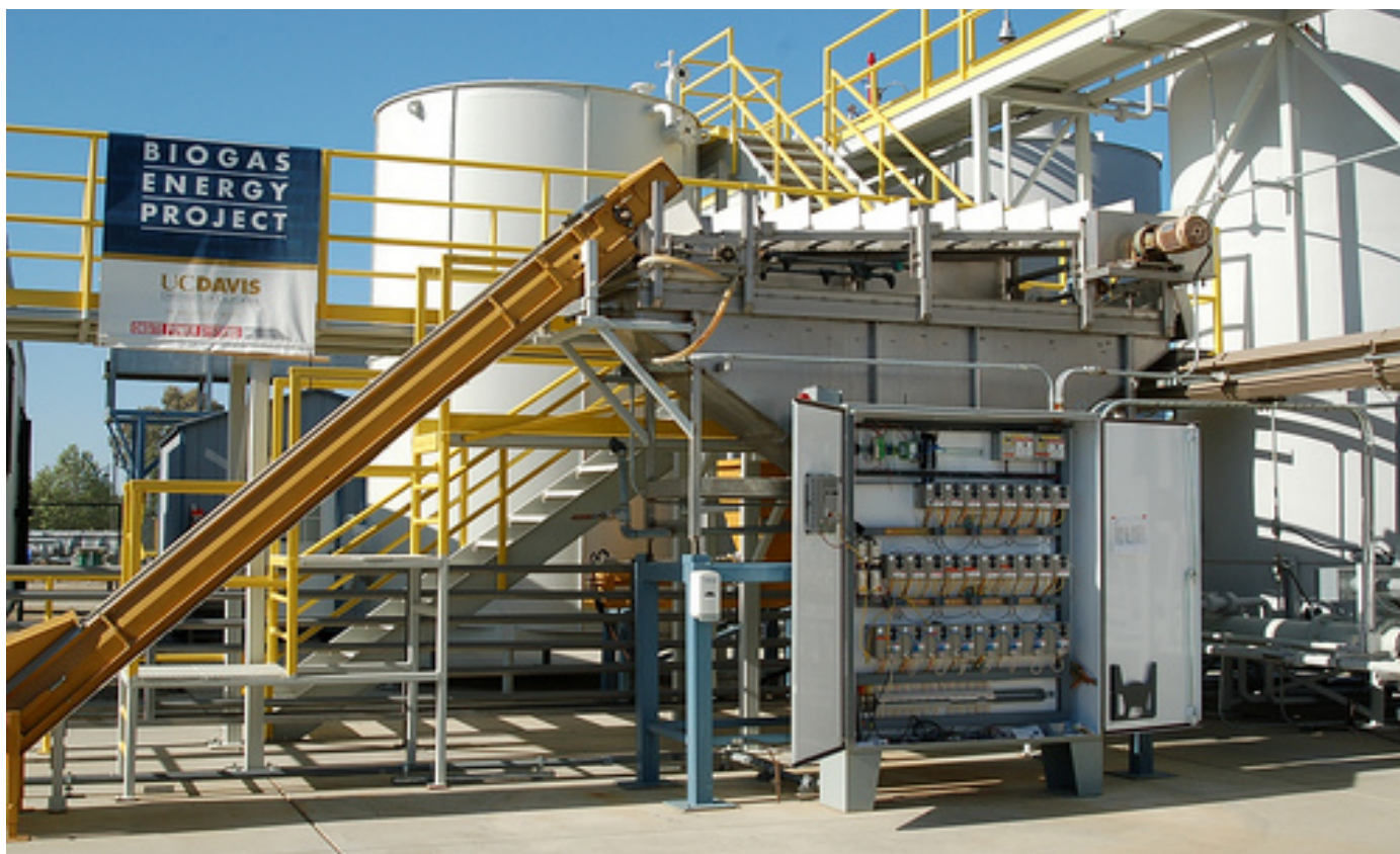
Figure E.5: Anaerobic Digester – UC Davis
