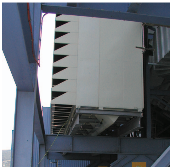
Figure 1. Gas turbine inlet with weather hoods
