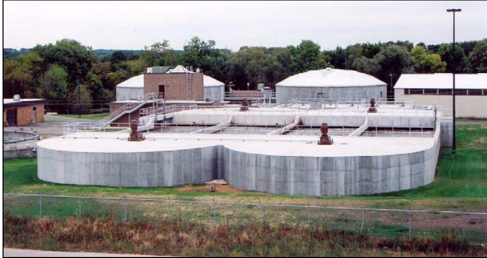
Figure 2 – Overview Picture of Ripon Oxidation Ditches
