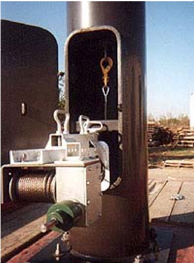
Figure 4.5: Typical high mast fixture lowering device
