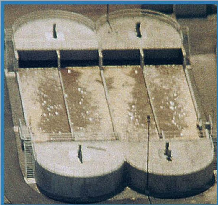
Designs utilizing common wall construction offer additional capital cost savings.
