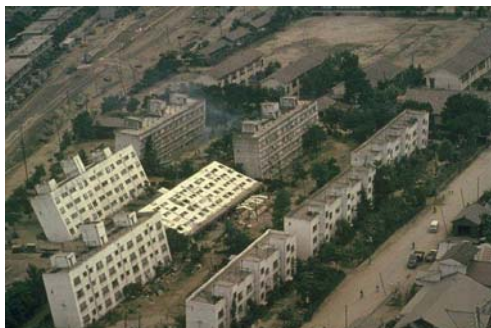
Figure 1.1: Buildings Destroyed by Liquefaction in Niigata, Japan, 1964
