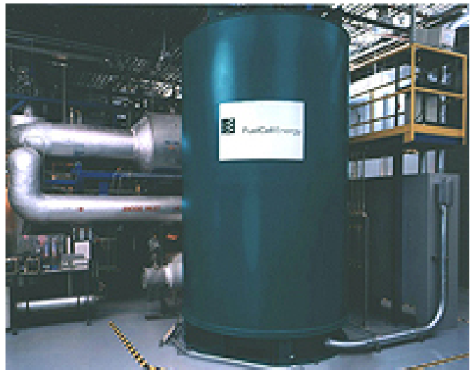
Figure 4.11: A Typical 20kW Commercial Application Fuel Cell Photo Source: National Energy Technology Laboratory, Department of Energy
