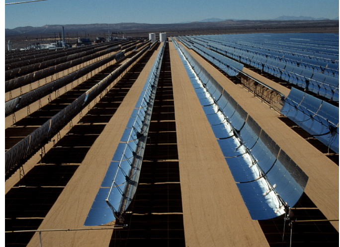
Figure E.3: Solar-Thermal Parabolic Trough Array
