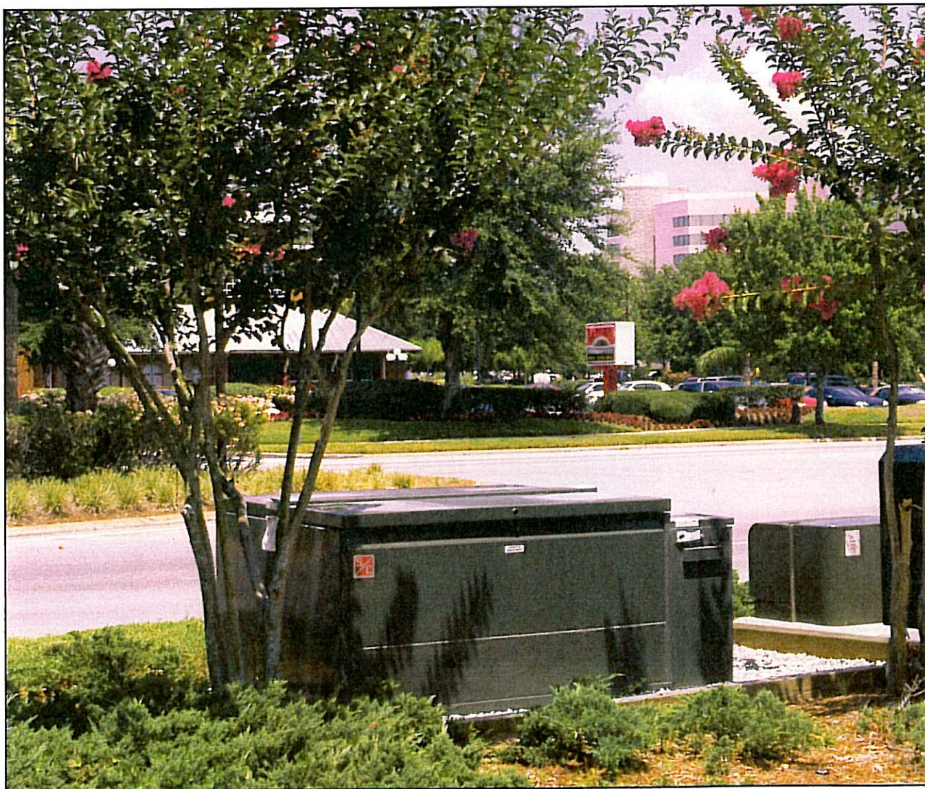
Remote Supervisory Pad-Mounted Style Vista UDS installation.
