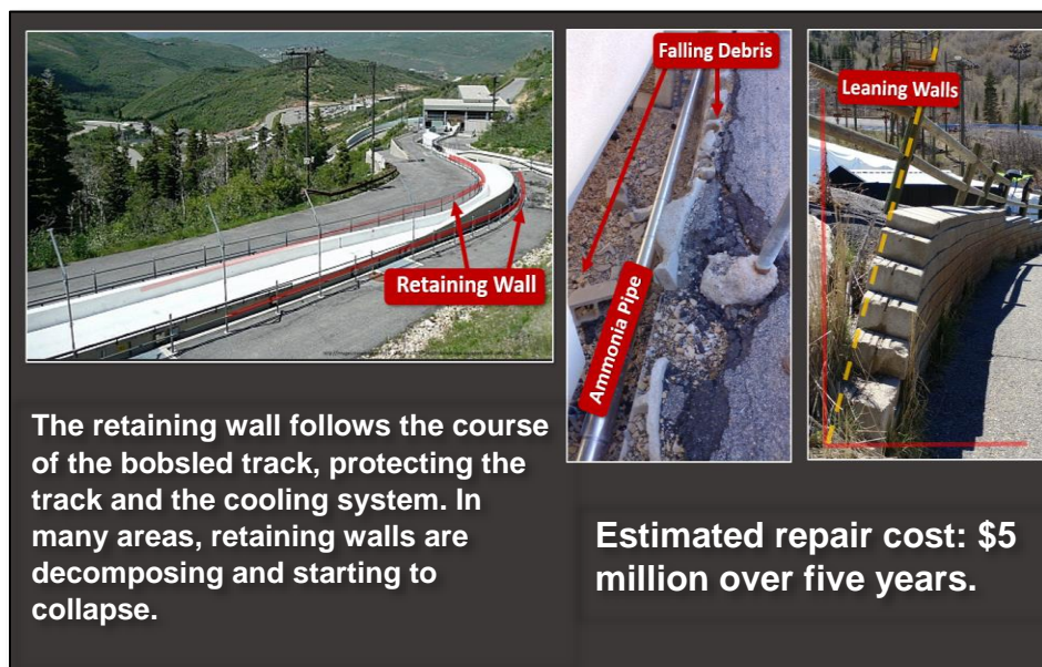
Figure 2.2 The Bobsled Track Retaining Walls Are Failing in Many Places. Retaining walls protect the track and the cooling system pipes that contain toxic ammonia gas as a refrigerant.
