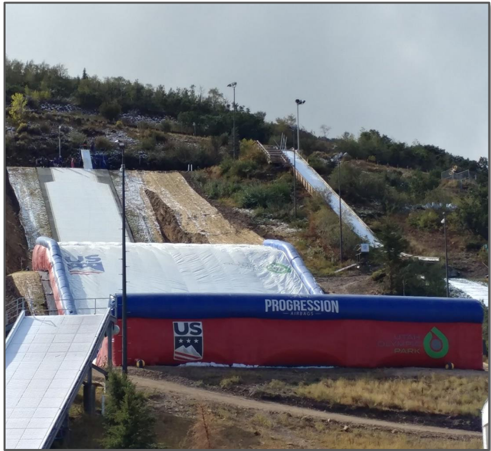
Figure 3.4 A New Freestyle Airbag Ski Jump Has Recently Been Built. An airbag allows freestyle ski jumpers to have a safe landing on a slope during the summer months.
