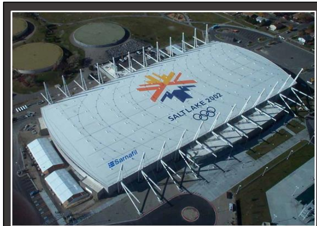
Figure 2.3 The Roof on the Utah Olympic Oval in Kearns Covers 4.5 Acres and Needs to Be Replaced. The original roof was expected to last fifteen years and now needs frequent repairs.
