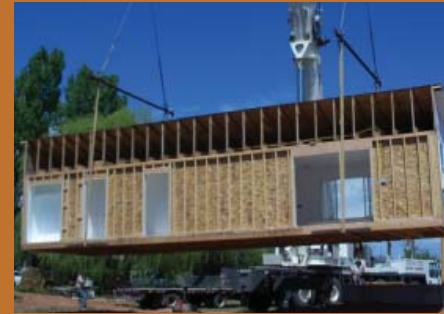
Home being assembled at the Justice Center
