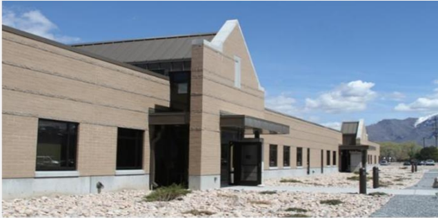
75 th Security Forces Building $7.1M Cost ($203/sf) Estimated MILCON Savings: 40-45%
