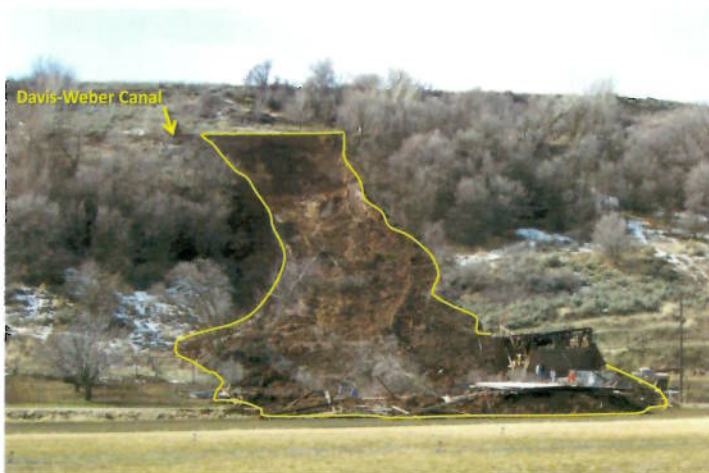
The 2005 landslide below the Davis-Weber Canal in South Weber, Davis County, that demolished a barn and covered part of State Route 60 (landslide outlined in yellow). The landslide occurred in one of the steeper parts of the slope composed of prehistoric landslide deposits that had been historically active.
