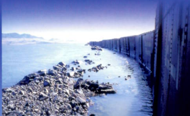
Boxcar seawall from the “seaward” side, September 1983, with berm on far left.
