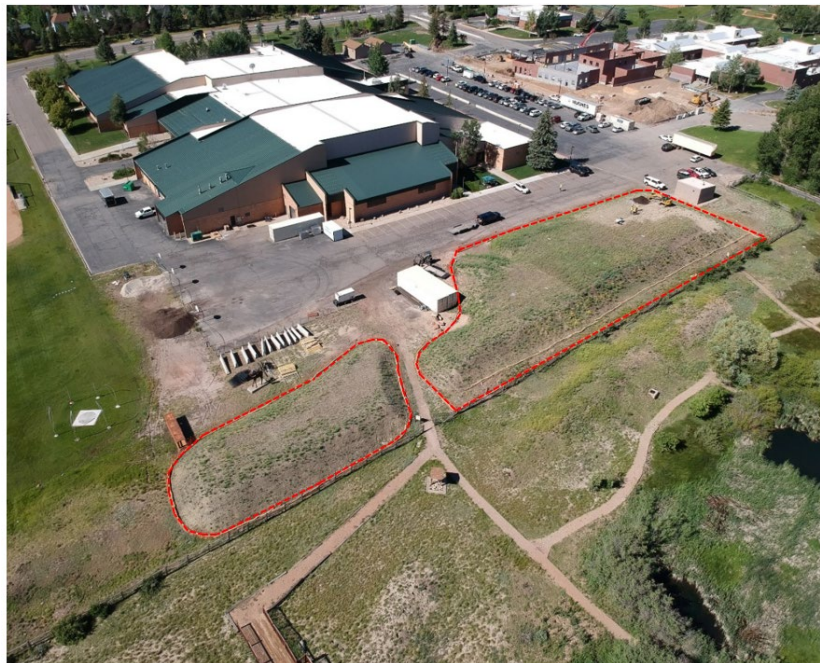
Figure 1.2: Waste Piles on the Junior High Property. The soil and the construction and demolition piles are situated just north of the junior high. We have overlaid red outlines to help differentiate the two piles.
