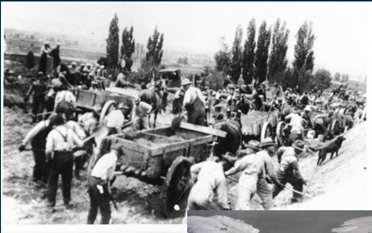
Left: Canal construction in Smithfield, courtesy of Katie Henrie.
