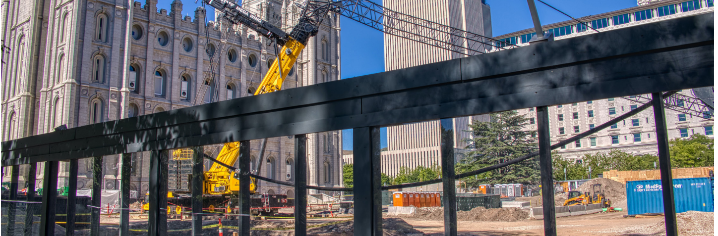
The Salt Lake Temple is currently undergoing a major seismic upgrade to prepare for the “Big One.”
