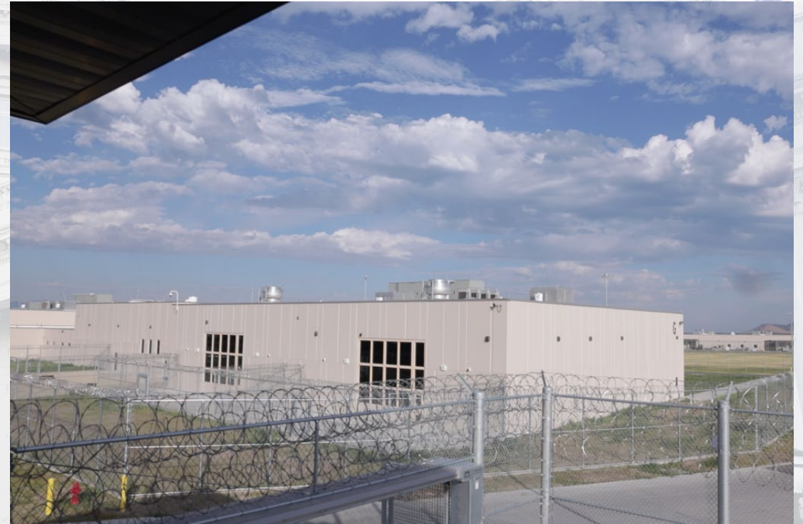
Photo of Utah State Correctional Facility from UDC Website
