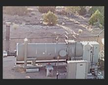
Oil, gas and saline water are separated in heater treaters.
