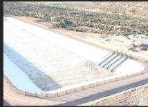
Saline water (~13k TDS) moves via metered pipelined to a lined holding pond.
