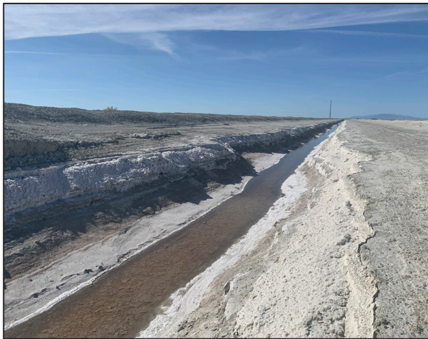
Brine extraction ditch (image by Jeremiah Bernau).
