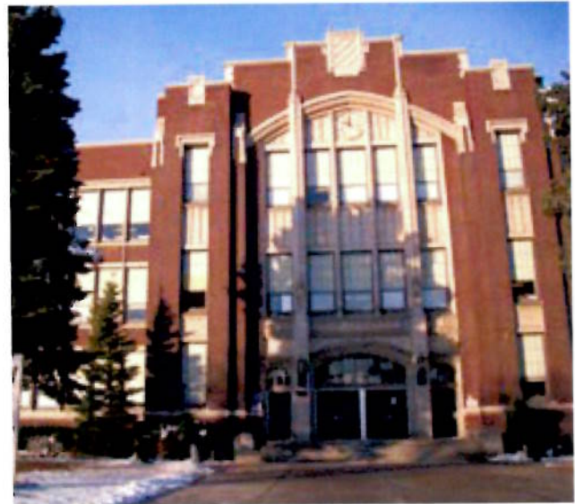
West High School is a URM school that was retrofitted in 1996.
