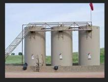
Saline water (~13k TDS) is stored in tanks on well pad.
