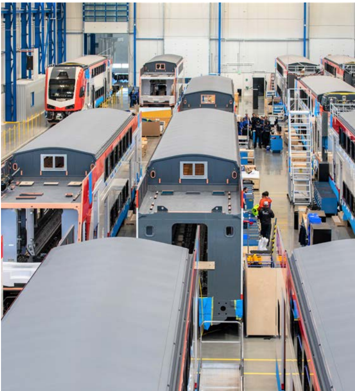
The Utah Inland Port Authority partnered with Stadler Rail US to fund a nearly complete test track at Stadler's Northwest Quadrant location, enabling the manufacturing and testing of electrified rail while providing public benefits such as job and training opportunities, enhanced rail access for local businesses, and preserved access to a vital rail corridor. —Photo Courtesy: Stadler Rail
