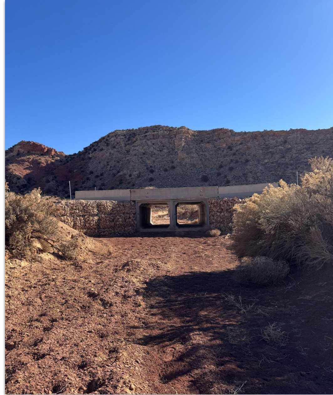
New culvert installation on House Rock Valley Road, Kane County
