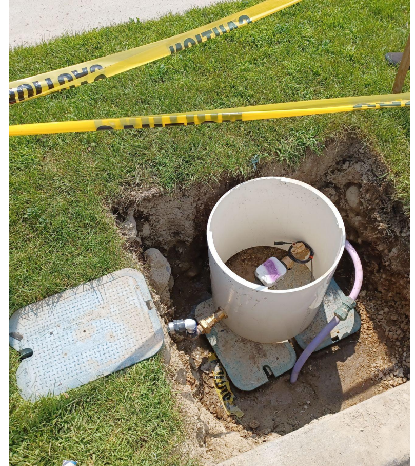
Secondary meter installation - Heber City
