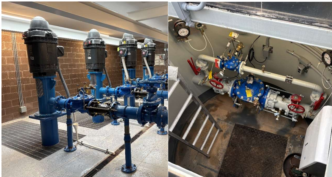
Figure 1 Pumps (Left Picture) and Valves (Right Picture) Move and Regulate Water Flow in Drinking Water Systems. These pictures come from a local drinking water system.
