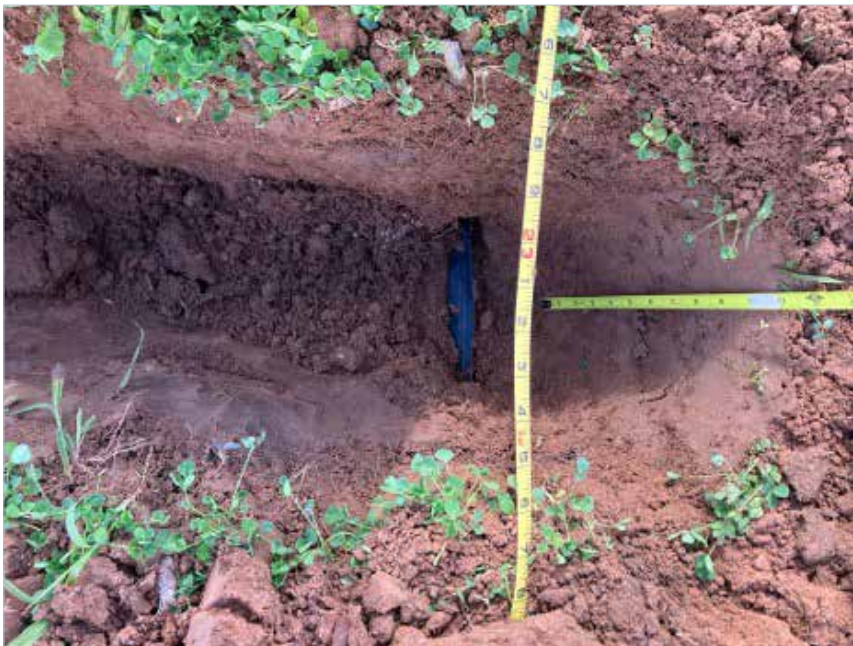
Figure 1: Subsurface drip irrigation line at the Pelican Lake pilot site.
