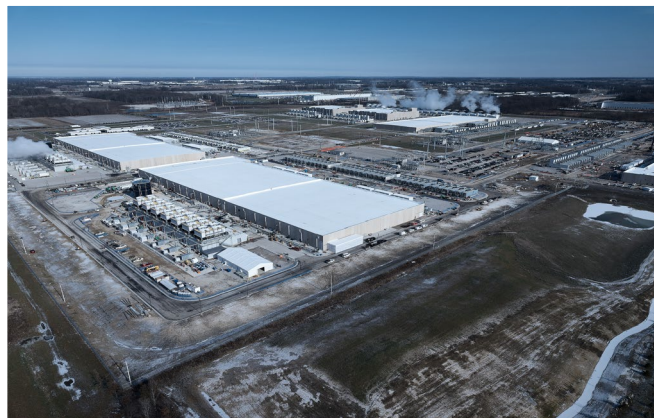
Aerial image of Google's 275,000 square-foot data center campus in New Albany, Ohio.
